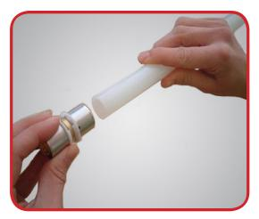
**2.** Insert the fitting into the pipe. The pipe must be seen through the check holes of the sleeve.
