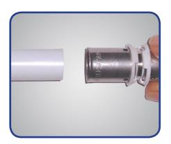
**3.** Insert the fitting into the pipe. The pipe must be seen through the check holes of the sleeve.
